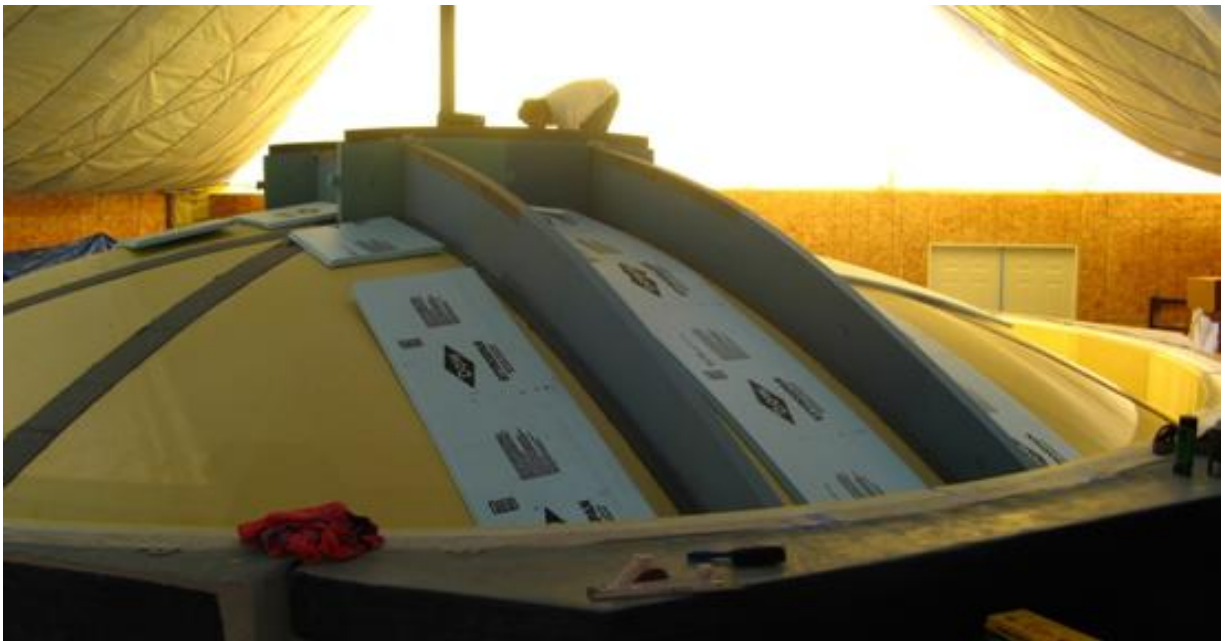
Figure 5 - The integrated structural beams are put into place.
