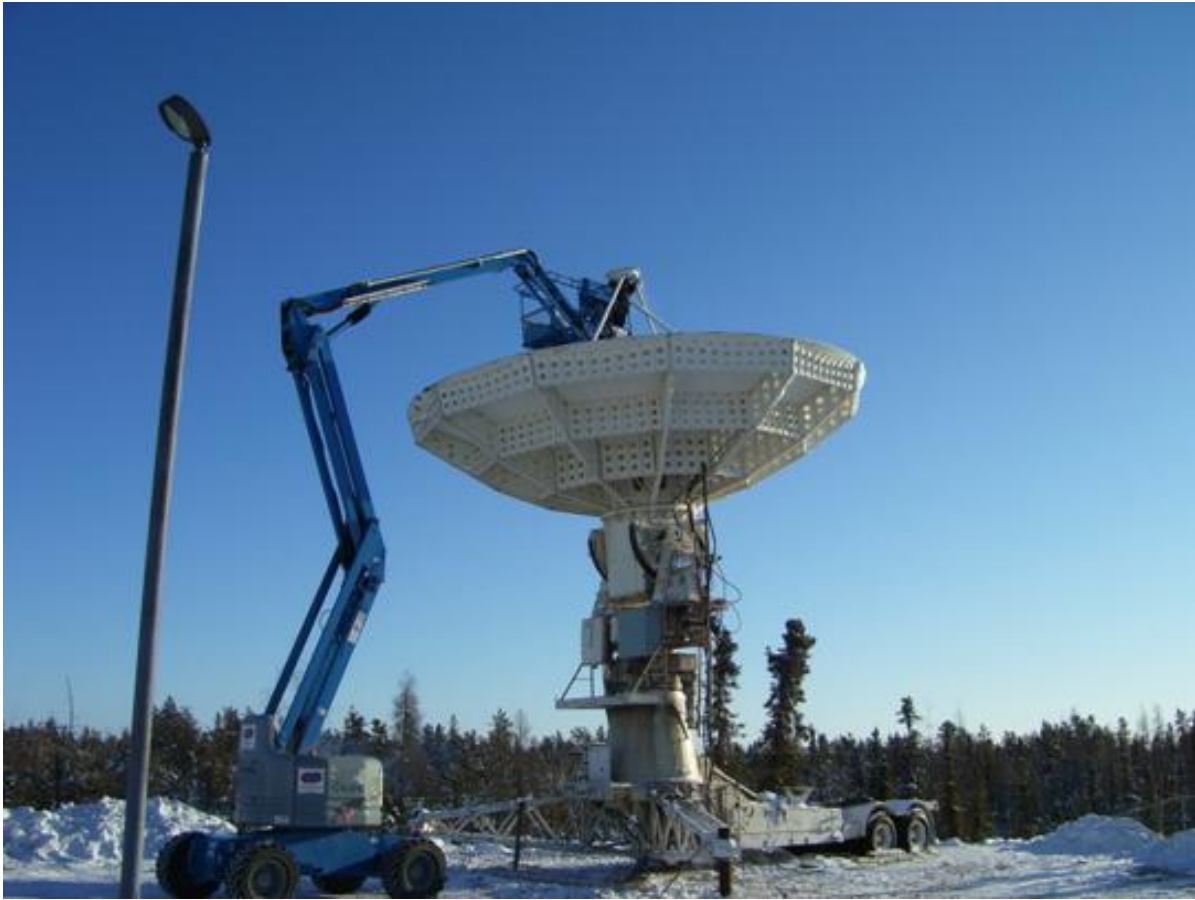
Figure 6 - The MV-1 antenna being disassembled in -30C conditions in Yellowknife. At least it was sunny!
