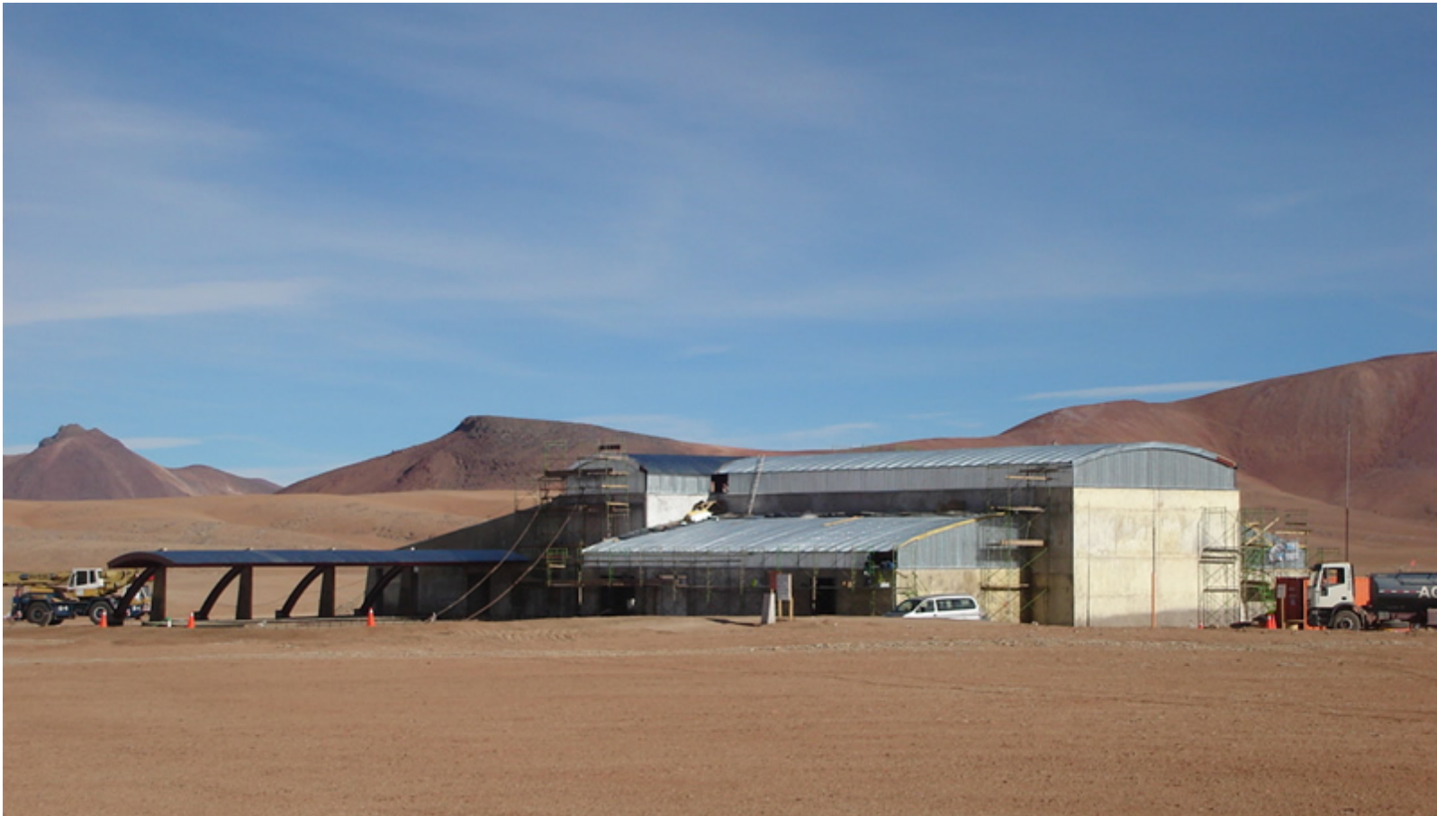
Figure 1: the completed shell of the main building for the Array Operations Center for ALMA at the high site (5000 m elevation)
